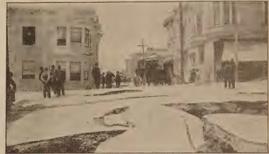
Great Fissures in the Street left by the Earthquake. The House on the Left Sunk to the Depth of one story into the Ground
